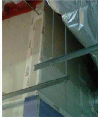
Proper wrapped corner
