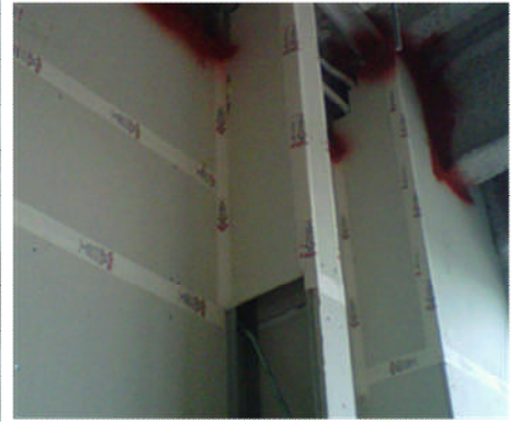
The double wrapped corner
